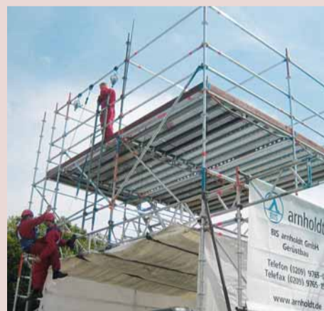
Evers demonstrating professional high-altitude rescues from BIS arnholdt scaffolding.
