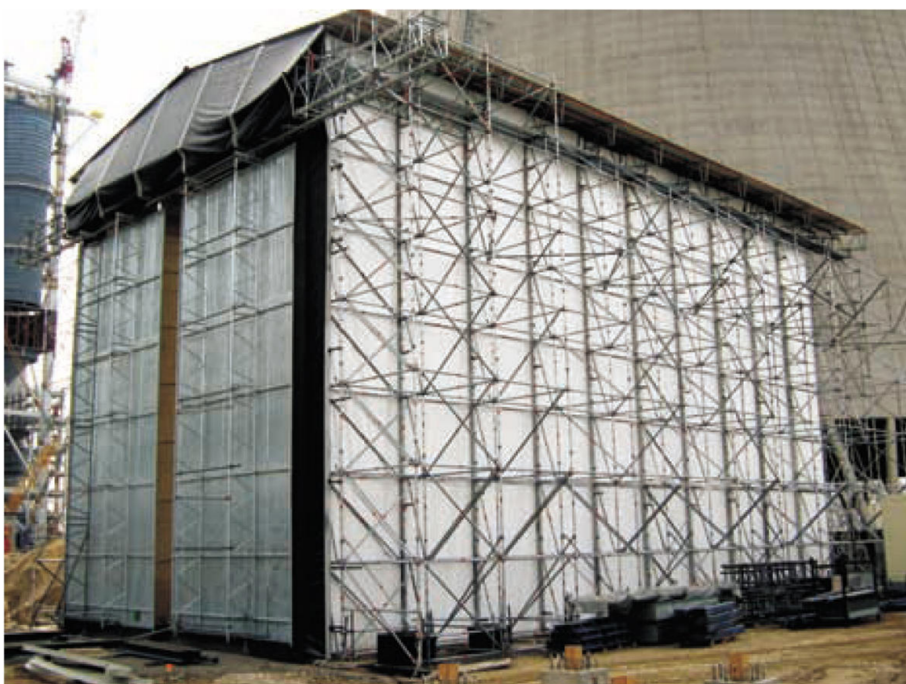
Project: temporary industrial hall at Bełchatów Power Plant
