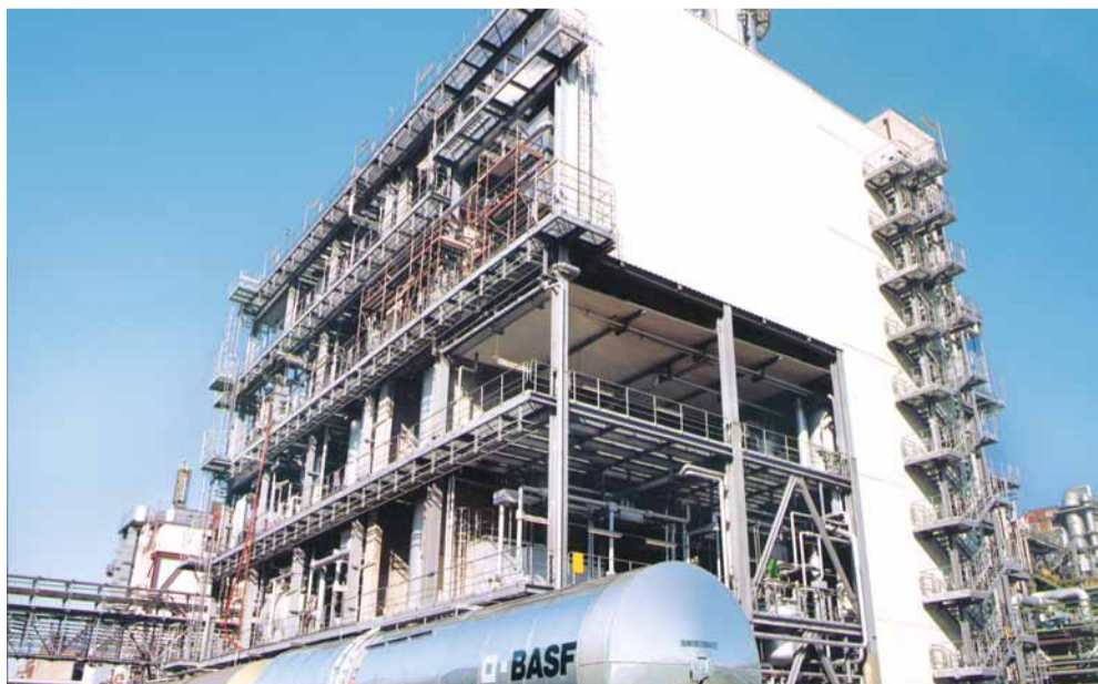
The planning of the pipework for a citral plant at BASF's Ludwigshafen location represented a challenging task for Peters Engineering.
